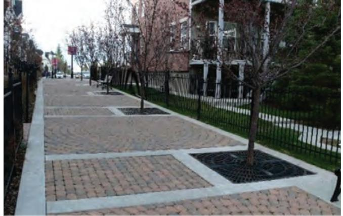
Figure 2.23: Pervious pavers with tree wells
